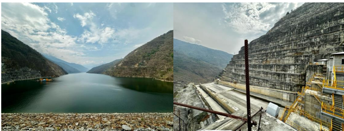
Figure 3.5 View from the Hidroituango dam to the Cauca River and tip of the infrastructure, Photo taken by Camila Botero, 2024
