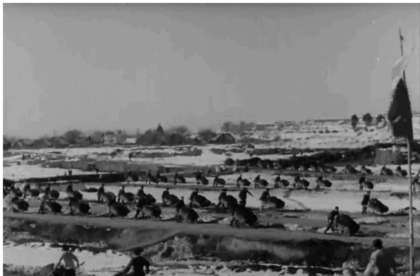
Fig. Xiashan Reservoir Construction 1 (Data Source: Sohu News)
