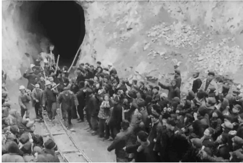
Fig. Xiashan Reservoir Construction 1 (Data Source: Sohu News)
