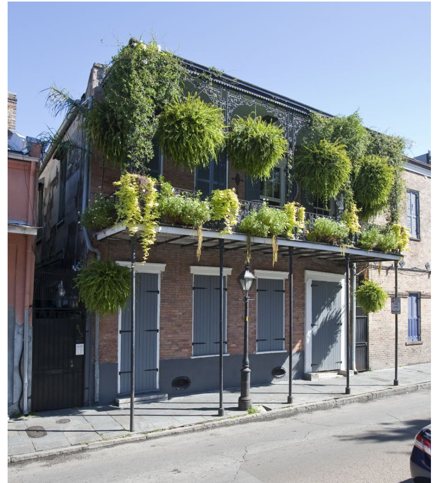
Figure 5.7: 813 Saint Ann Street (2020) Photograph by Caitlin Rudin Gardenhire
