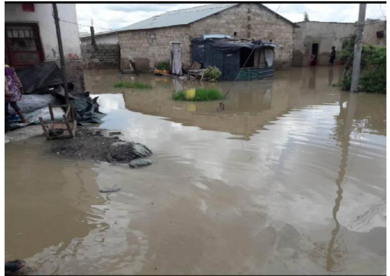
Figure 1: Flooding in an unplanned settlement in Lusaka Photo by Wilma Nchito (2017)
