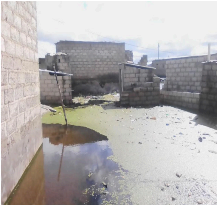
Figure 2. Abandoned housing due to flooding Photo by Wilma Nchito (2017)
