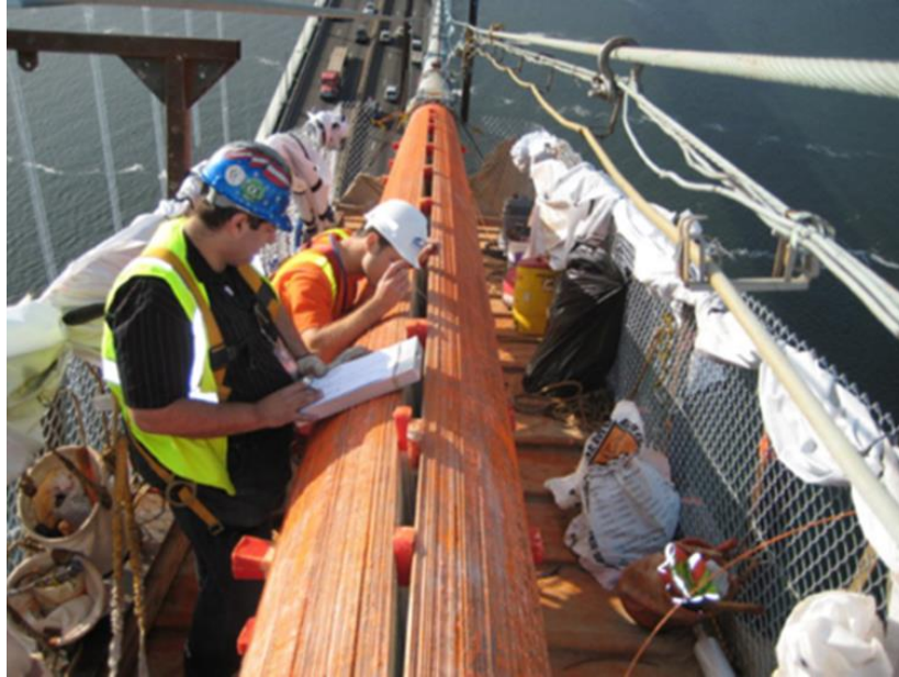
Figure 2.1: Inspection of a suspension bridge main cable using wedging (courtesy of Modjeski and Masters).
