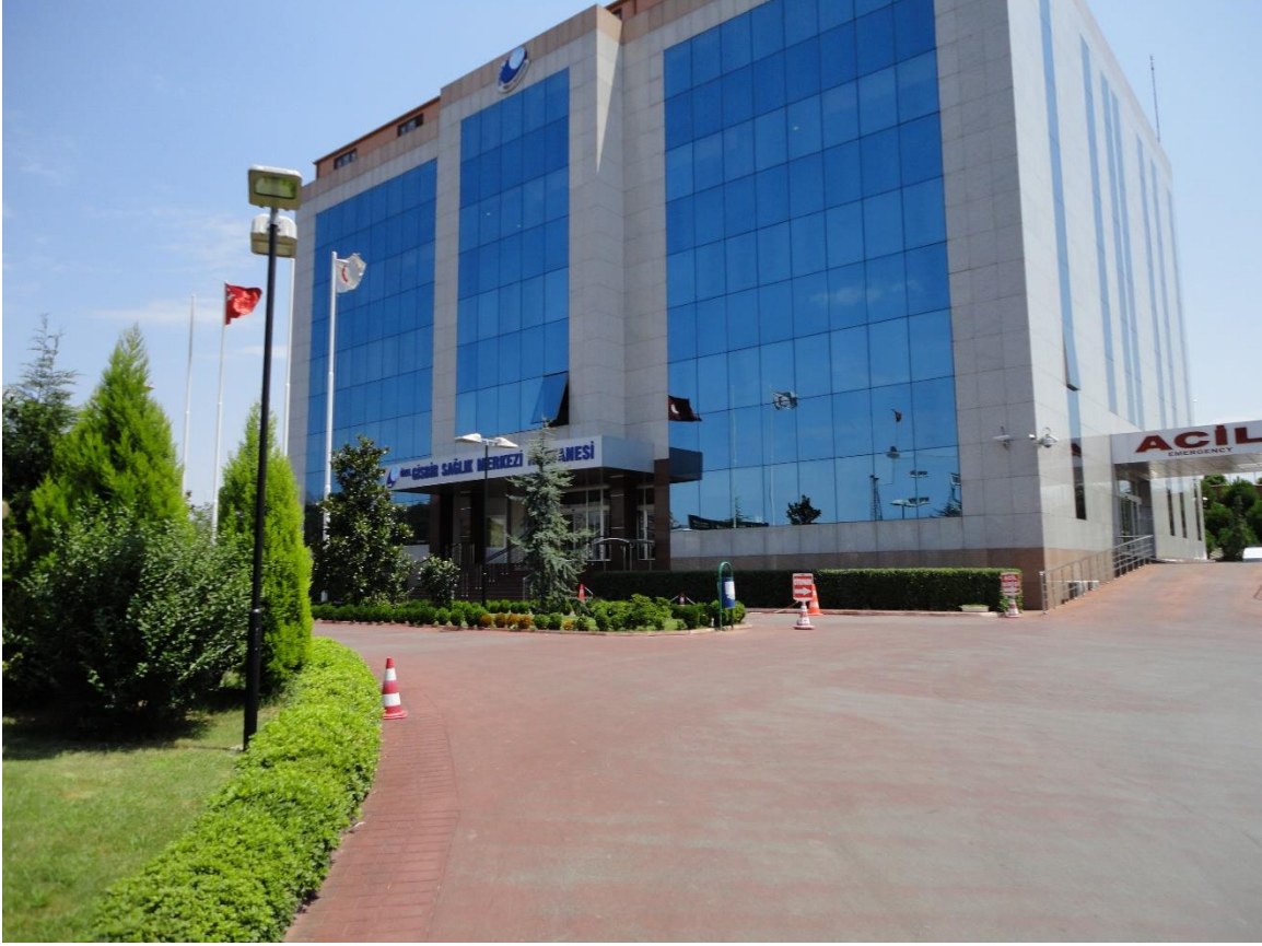
Figure 12: Tuzla Shipbuilders Association (GİSBİR) Private Hospital. The hospital is located across the street of the chain of the shipyards in Tuzla. The entrance of the emergency service (ACİL) is directly connected to that main street, so that injured workers can be brought to hospital quickly (photo taken by myself).
