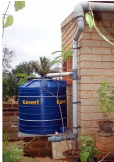
Figure 3: Basic system design; a basic rainwater harvesting system, such as the one pictured above, can be built of basic materials for the equivalent of $60, depending on local costs and system size; the main technical requirements are an impervious roof and room for a cistern or tank (Photo: S. Vishwanath, Rainwater Club).
