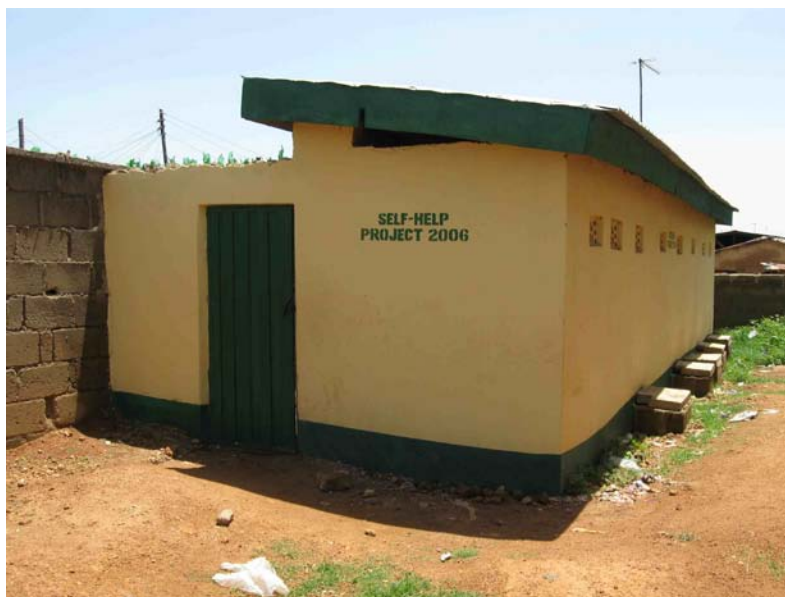
Figure 7: Photo of Toilet Block Constructed in 2006
