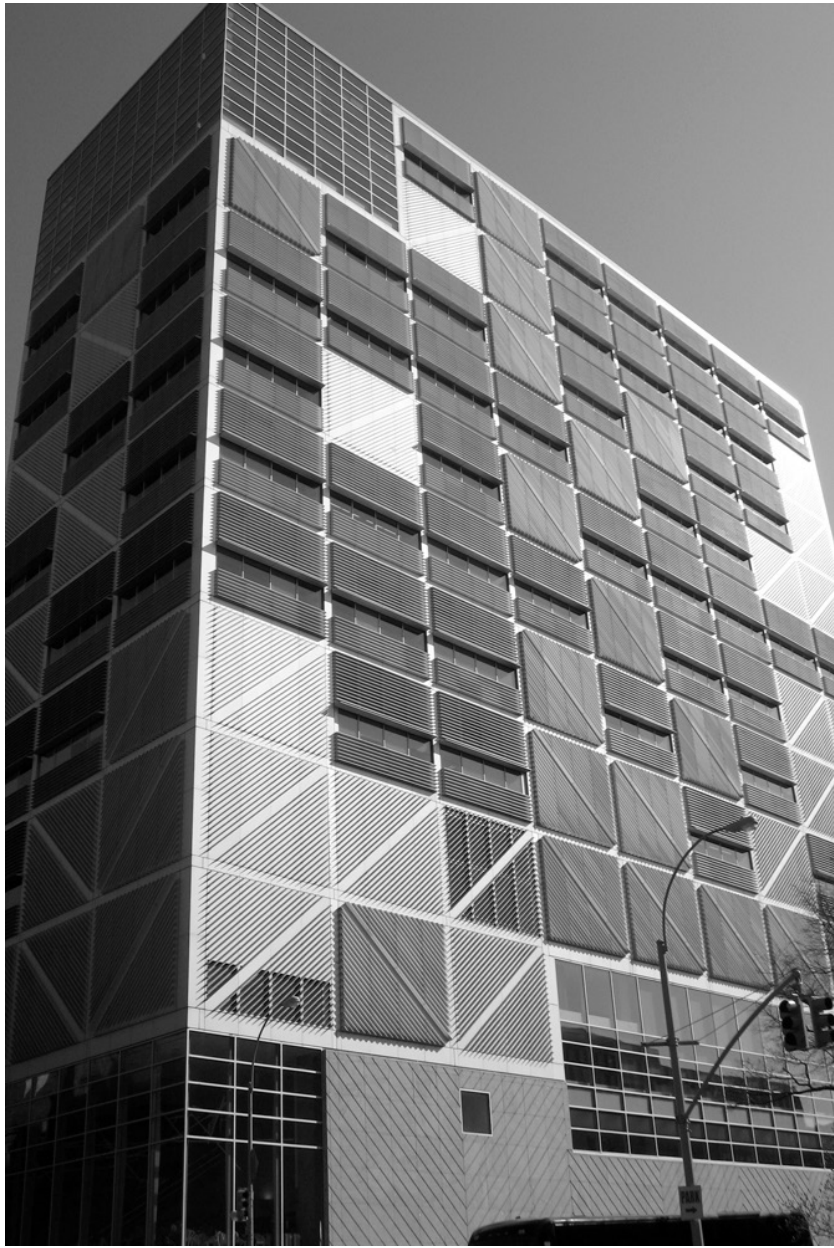
FIGURE 7.2 The Exterior of the Northwest Corner Building
