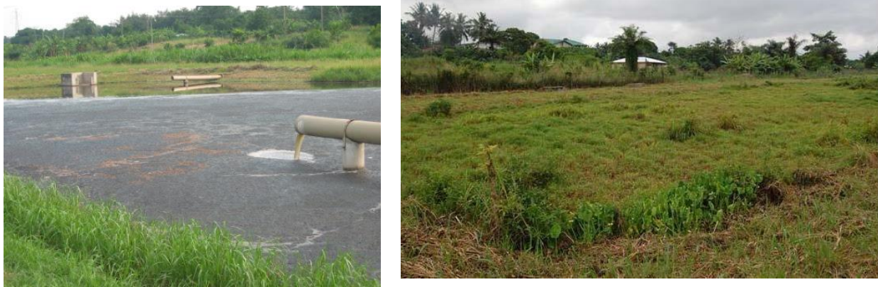
Figure 7. Treatment Plant at Asafo and Overloaded Anaerobic Pond at Ahesan
