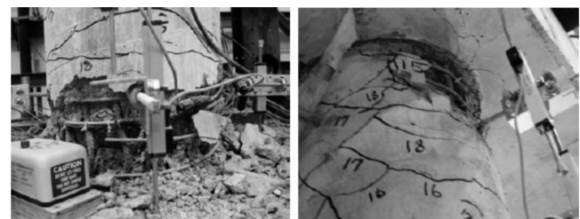
Fig. 3. Damage observed on the lower and upper portions of Bent-3 after T-19
