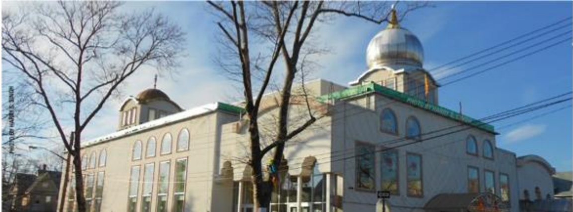
Figure 6. A re-built Sikh Cultural Society Gurdwara after a fire in 2003 destroyed the original building
