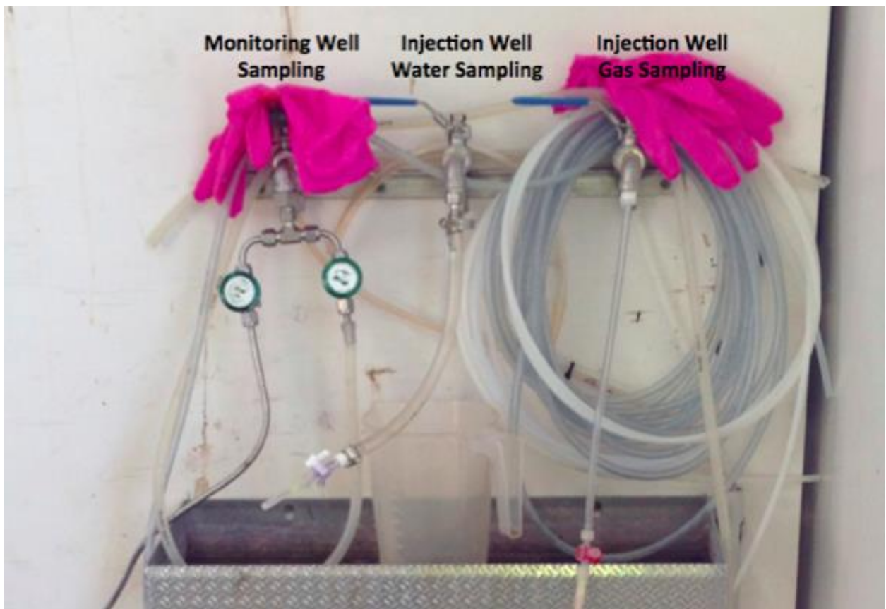
Figure 44: Surface water sampling ports in a hut before HN-2 in field test.
