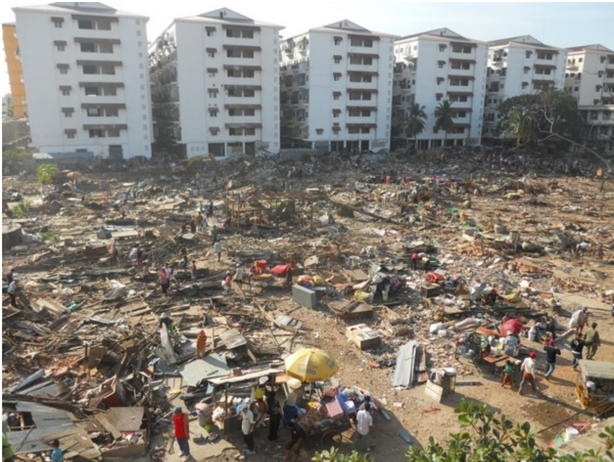
Site of Borei Keila settlement during demolition phase
