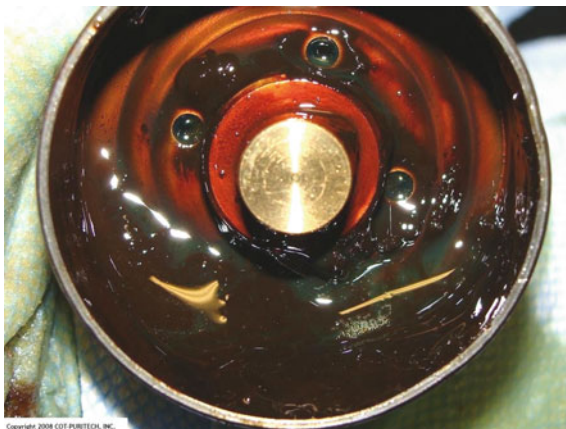
Fig. 18.27 Water-induced additive drop-out fouling a gearbox thermostat, rendering it inoperative (COT-Puritech, Inc.)
