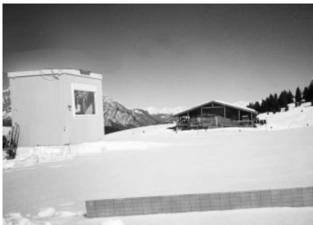
Fig. 2. The microwave station.
