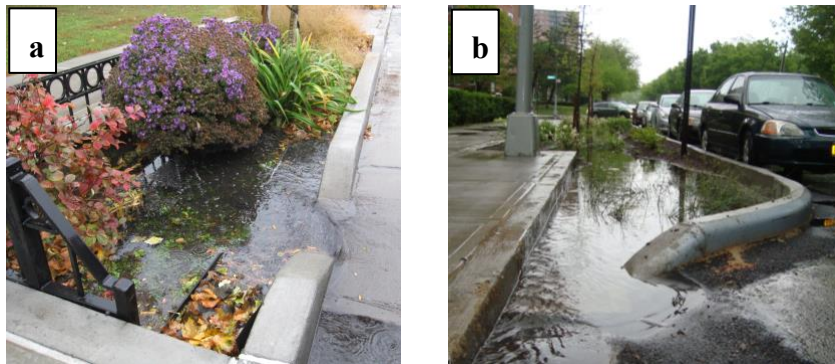
FIG. 2. Bioretention study sites: Right-of-Way Bioswale (a) and Stormwater Greenstreet (b)
