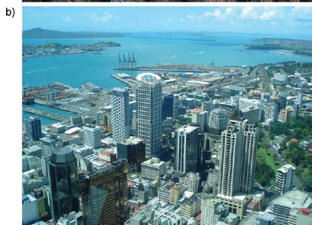
FIGURE 2. Higher density and population, combined with an aging, unsustainable infrastructure, will mean that New York City (a) will require long-term funding, planning and engineering to transition to a sustainable infrastructure. Auckland (b), with a younger infrastructure and lower density and population, will need to consider new types of infrastructure and resource management to ensure it embeds a sustainable infrastructure as it continues to grow.
