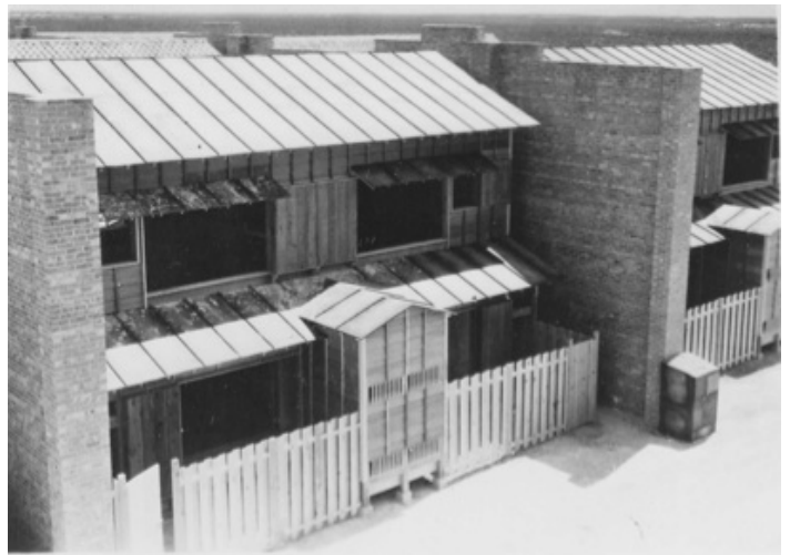
Typical Unit Between Fire Walls
