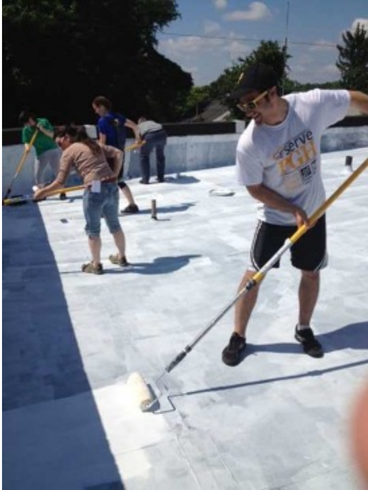
Volunteers apply reflective white paint at 7024 Lemington Ave
