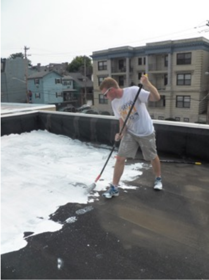
Volunteer applies reflective white paint at 259 McKee Pl
