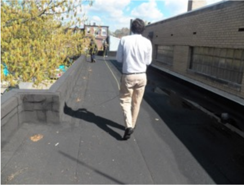
Program administrators measuring roof dimensions at 1124 North Avenue
