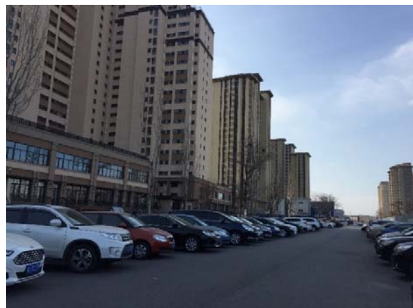
Figure 14 Main parking area at the north side.
