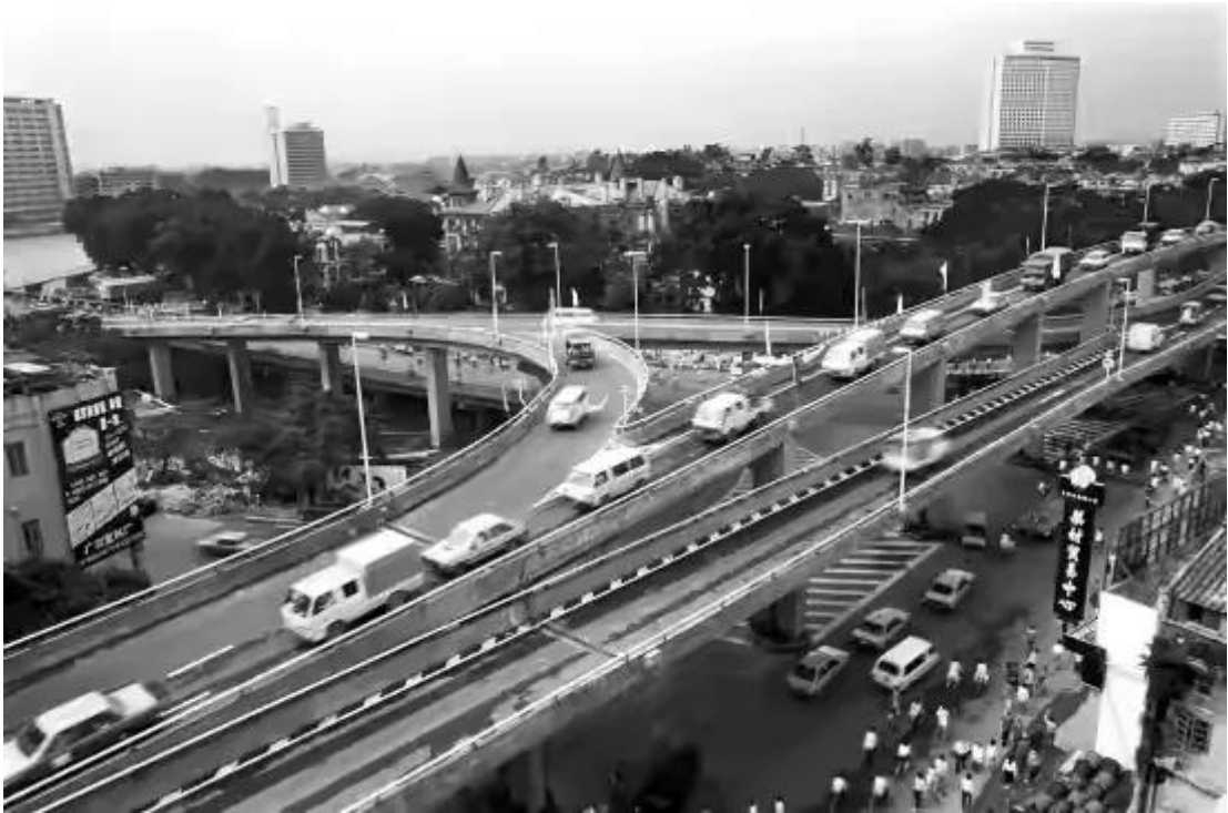
Fig 3-1 Renming Road Viaduct: the first urban viaduct in the country
